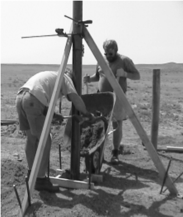
Setting an array pole in concrete.
