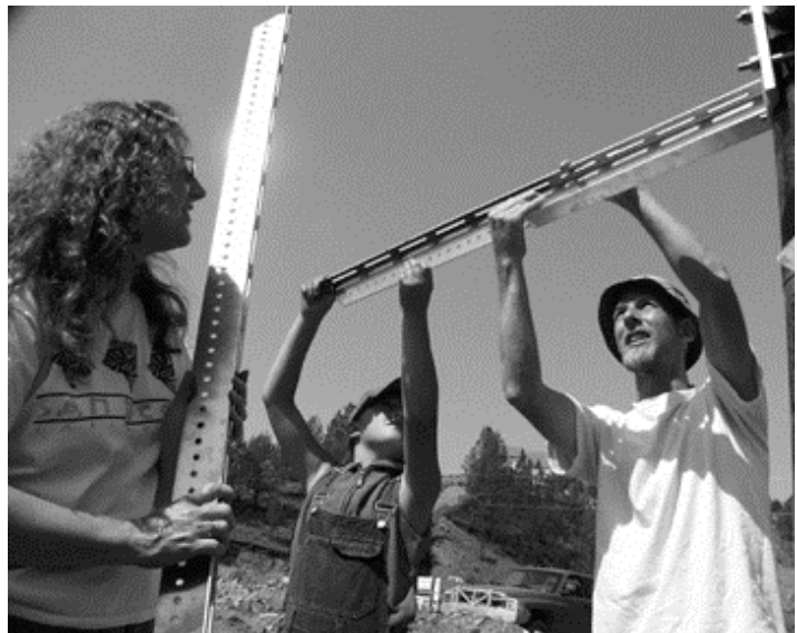
ETA-300 PV array assembly The mounting pole is short enough to facilitate assembly without mechanical assistance.
